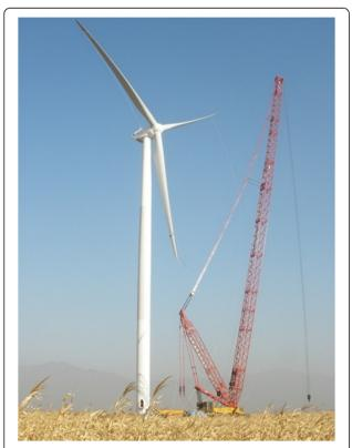
Figure 3 The 2.5-MW Goldwind PMDD wind turbine during erection.
