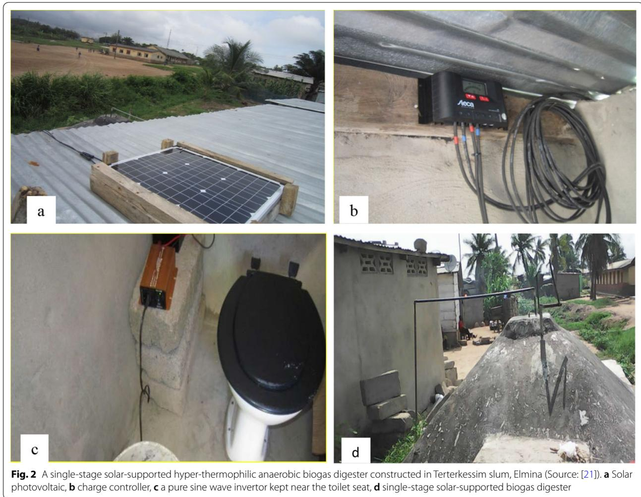
hyper-thermophilic anaerobic reactor for biogas production and disinfection of BW in the Terterkessim slum, Elmina-Ghana (Fig. 2). A Household-Based Survey (HBS) was conducted in 2016 to assess the perception of residents in Elmina-Ghana, on their willingness to adopt the SSHTABD in their homes if it was constructed for them.
